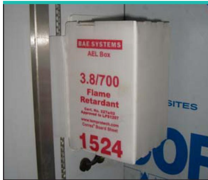
Figure 8.4 AEL Protection Box as Fitted
