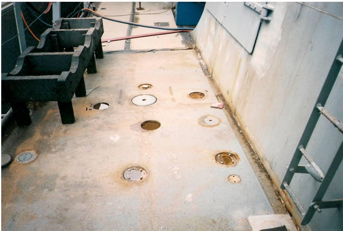
Figure 3.6 Generic Deck Connection Issue
