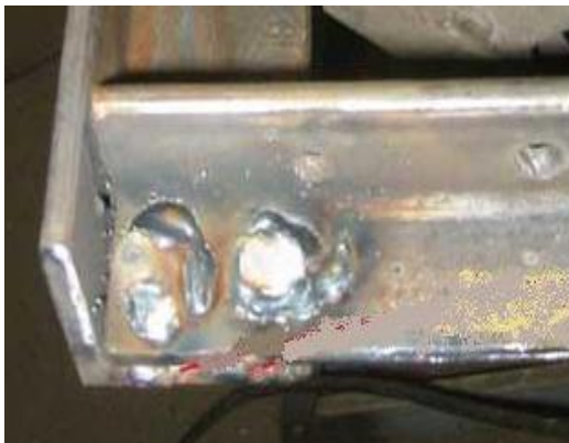
Figure 3.12 Open Tack Weld
